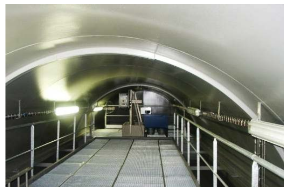
Inside view of the technical dome
