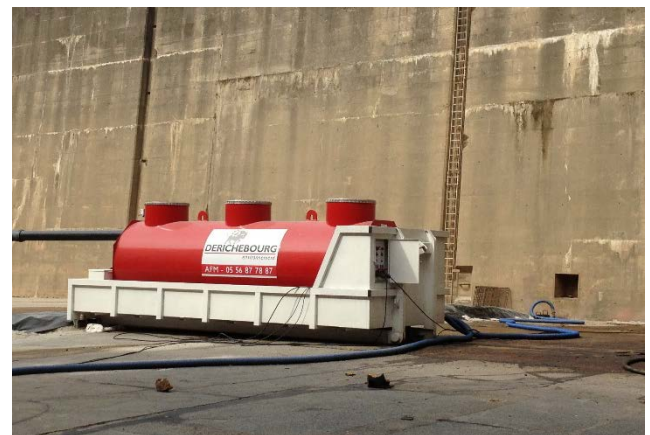
Installation on a mobile storage wagon
