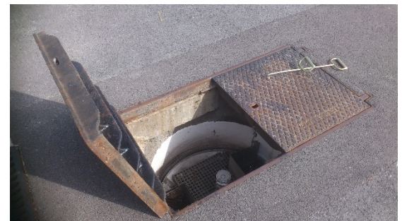
Installation under the road with full access
